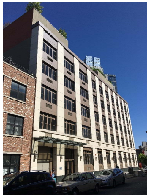
VIEW OF COMPLETED SOUTH-EAST BUILDING FAÇADE ALONG KEAP STREET
