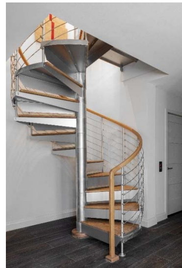
STAINLESS STEEL SPIRAL STAIR CONNECTING TO KITCHEN ABOVE
