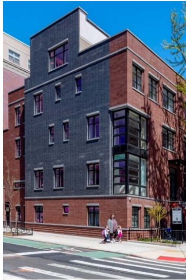
PARTIAL VIEW OF 311 STATE STREET CORNER TOWNHOUSE LOOKING NORTH EAST
