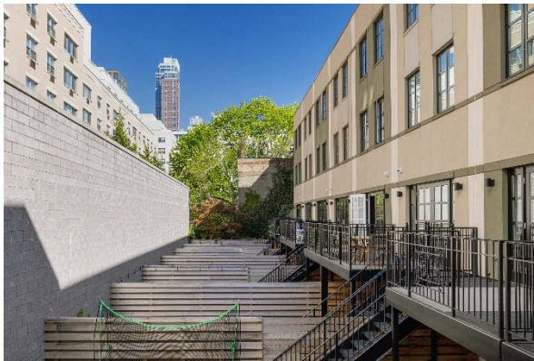
NORTH FAÇADE WITH EIFS SYSTEM
