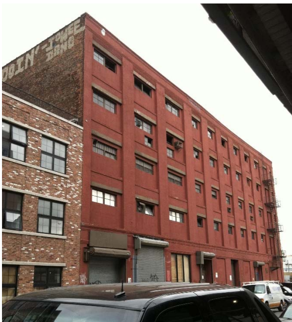
EXISTING SOUTH-EAST BUILDING FAÇADE ALONG KEAP STREET BEFORE CONSTRUCTION
