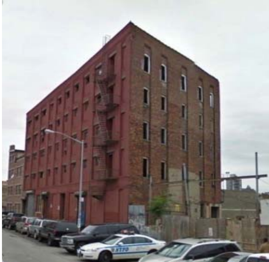
EXISTING NORTH-EAST BUILDING FAÇADE ALONG KEAP STREET BEFORE CONSTRUCTION
